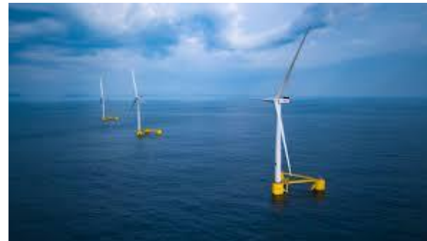
Above: The 50MW Kincardine Floating Offshore Wind Farm 15km off the coast of Aberdeen, fully operational in 2021. Image courtesy of Principal Power
